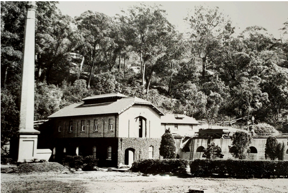
Then: The sewerage works in about 1898 showing the chimney, engine house, septic tanks and sand filter beds in foreground
