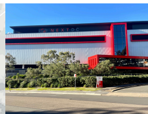
NEXTDC Sydney Data Centre, Macquarie Park.
