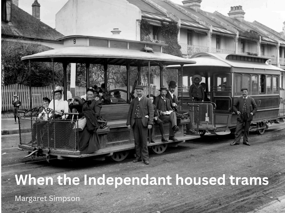
North Sydney cable tram set showing a grip car in the foreground and a trailing car in the background at St Leonards c.1893. Photo by Arthur Phillips.
