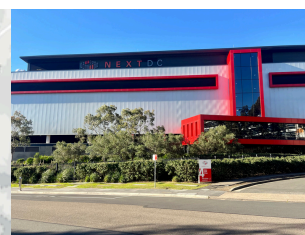
NEXTDC Sydney Data Centre, Macquarie Park.
